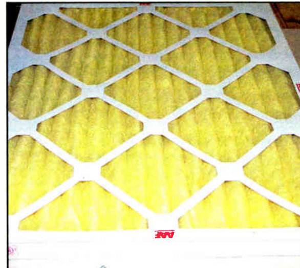
Fig. 3: Mark high-efficiency filters with the date.
