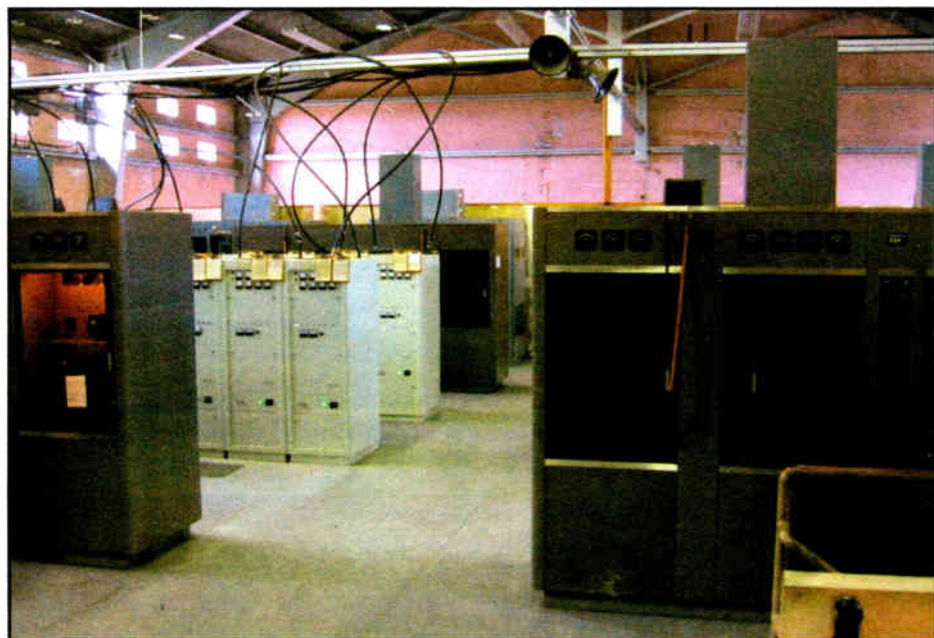
Upstairs transmitter gallery showing vintage RCA transmitters and more modern Henry units.
