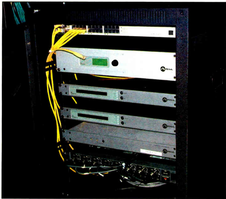
Axia system in place at NewCap Radio installation in Edmonton, Alberta.
