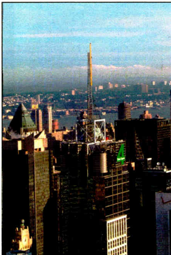
An ERI gin pole sits atop 4 Times Square in New York City.
