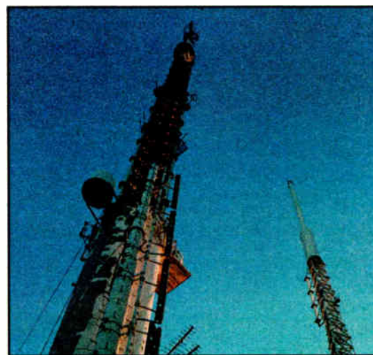
A view from atop the John Hancock Center includes an FM master antenna plus WBBM(TV/DT) at left, with more TV at right.
