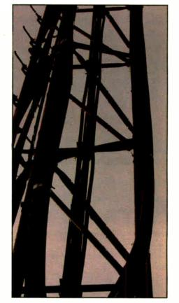
Fig. 2: Don't let coaxial cables obstruct the red and white painted tower legs.
