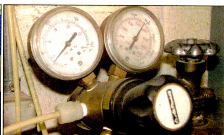
Fig. 3: Burn the hose off the tank, it becomes a fire extinguisher.
