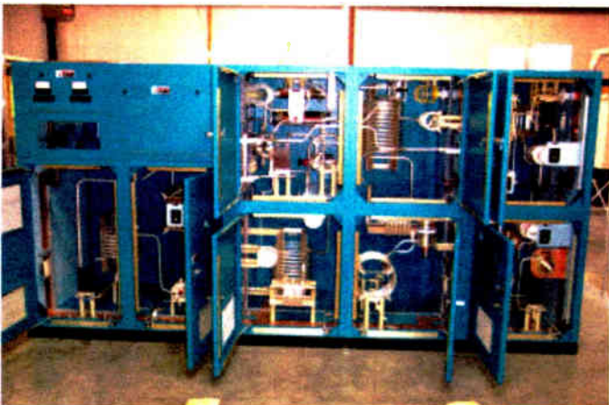
THREE TOWER AM 50kW NDA-D / DA-N DIRECTIONAL ANTENNA SYSTEM ST PAUL, MN.
