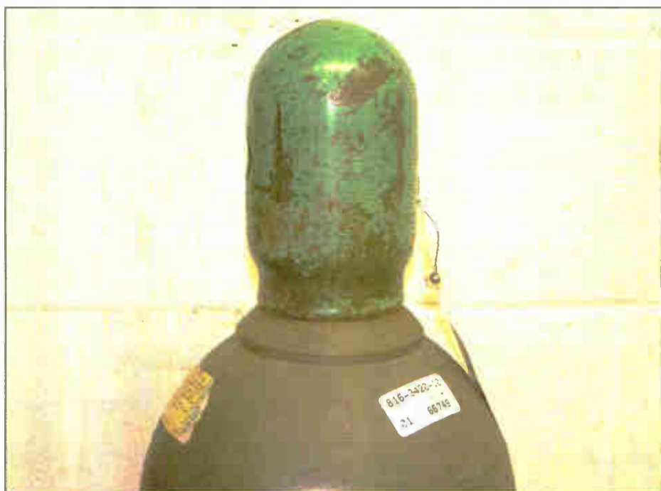
Fig. 1: Keep nitrogen tank caps secured to tanks that are not in use.
