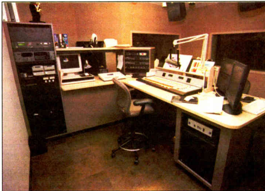
Studio Technology West provided Entercom with an ergonomic furniture design and solid-surface countertops.
