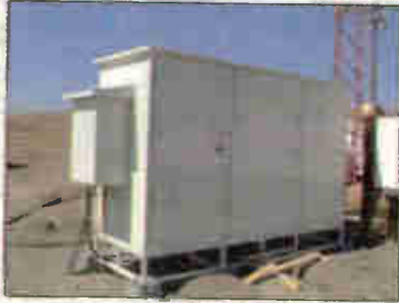
KAFY Radio Bakersfield, Ca 3-Tower 1/5kW DA-2 970KHz
