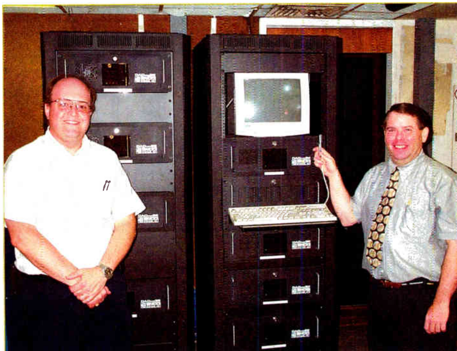
Tom Ray, left, and Kerry Richards pose with the ENCO servers.
