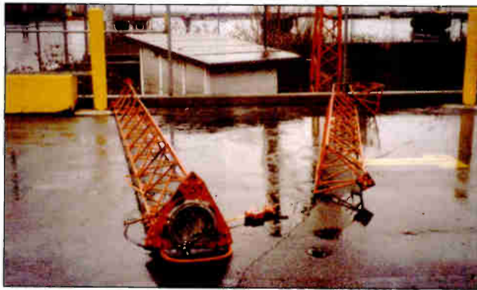
Shown are two sections of the top 40 feet of KJR(AM)'s tower after being lowered by riggers.
