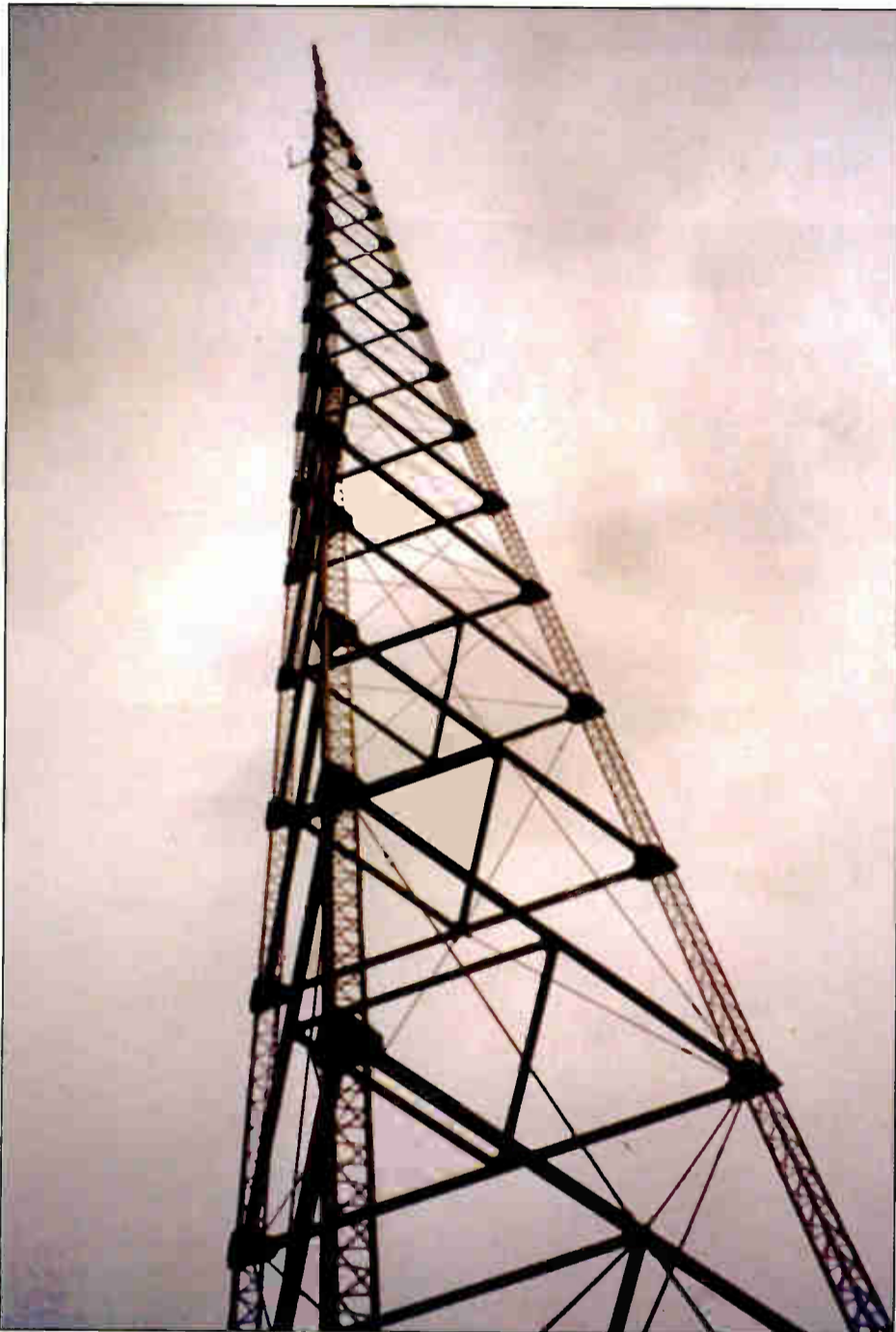
The KJR(AM) Tower, Missing Its Top Sections
