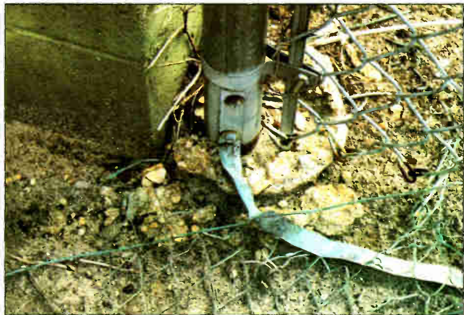
Fig. 4: Grounding the fence at an AM tower site
