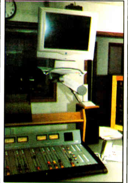
Fig. 3: A heavy-duty monitor stand that raises the monitor to eye level, if needed
