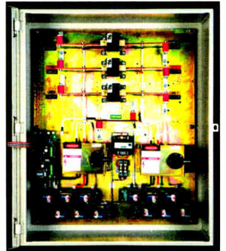
Internal View of the Model SDX
