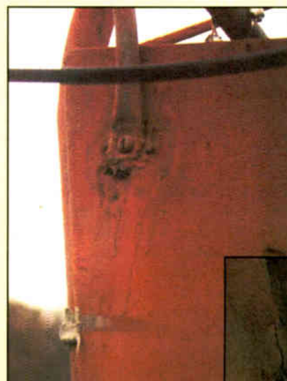
Fig. 4: Check towers for loose connections, rust and corrosion.
