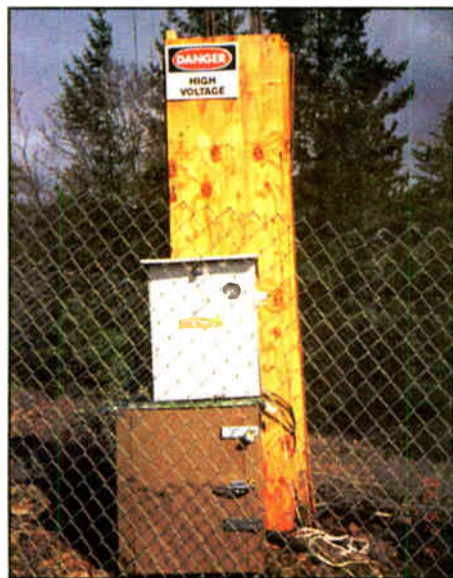
It appears the ATU is stationed on top of an old refrigerator.
