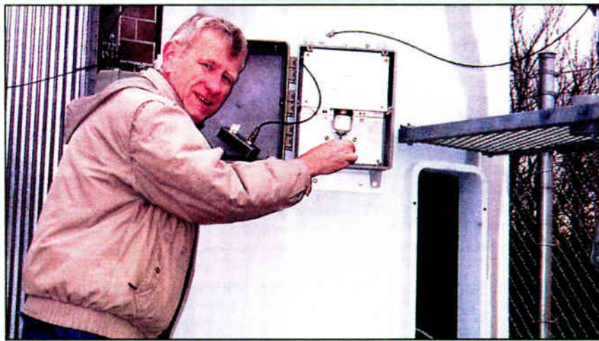
Larry Waggoner at the Cellular One Tower in Wichita, Kan.
