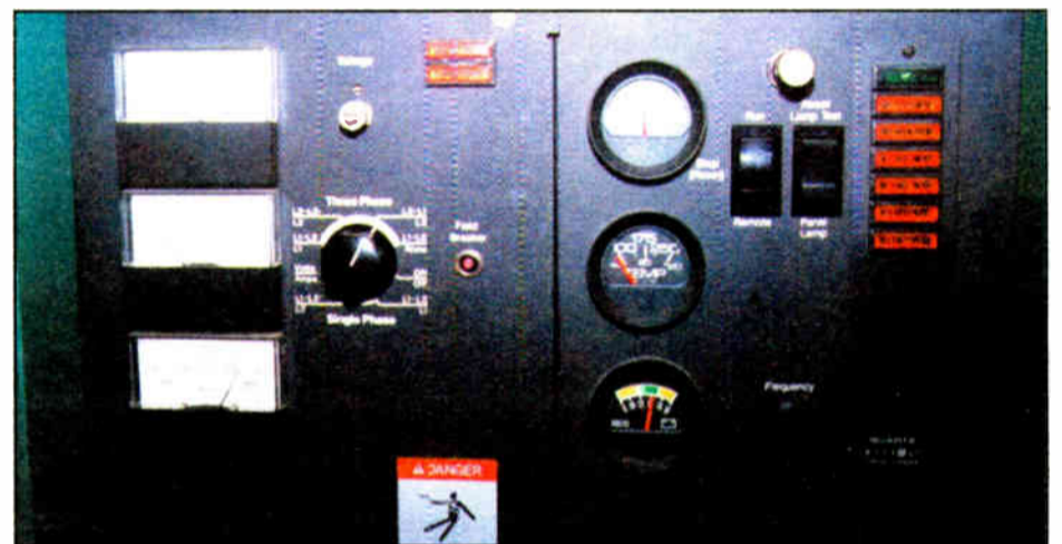
Figure 1: Take periodic meter readings of your generator, as well as your transmitter.
