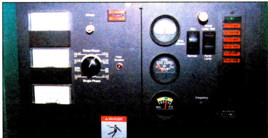
Figure 1: Take periodic meter readings of your generator, as well as your transmitter.
