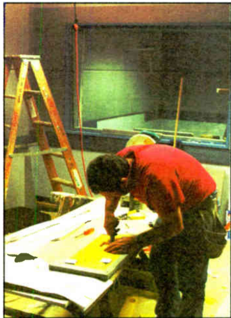
At Work on the New Studios
