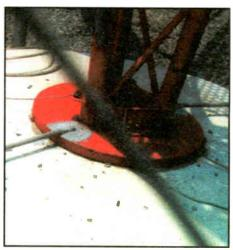
Figures 3 & 4: Left: RTV compound plugs the entrance of this PVC pipe used to protect ground wires. Right: The PVC pipe also works well at the base of a tower, protecting ground wires.
