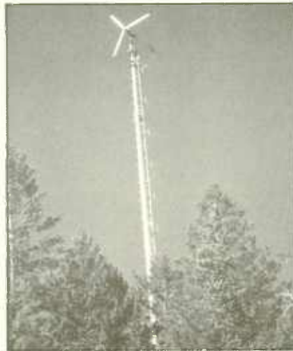
Powered by an alternative energy source, the KFMU-FM tower in Oak Creek, Colo., rises above the trees.
