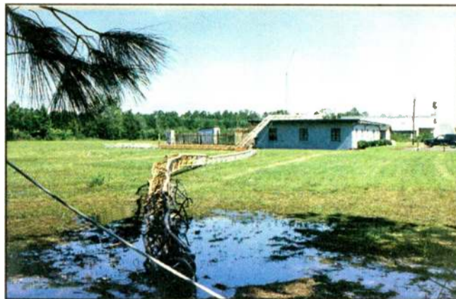
Fran Damage at WBLA(AM)-WGQR(FM)
