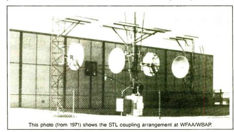
Enter Cullum's STL isocoupler. Explained Beavers, "The (STL-) coax goes down the tower to almost the base of the tower, stops and then hooks up to another dish. That dish is looking out toward yet another dish on a small little tower that is not fed with RF." The small tower is what Cullum used to isolate antennas from the two stations' STL feeds.
