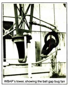
between what Kirk describes as cannon balls, which are attached to steel rods. One steel rod is attached to the tower and another is spiked into the ground near the base of the tower. The spark gap is a little over an inch wide, according to Kirk's estimation. Enough for a lightning strike to jump the gap and become grounded.
