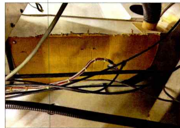
Covering the hole in the duct.
