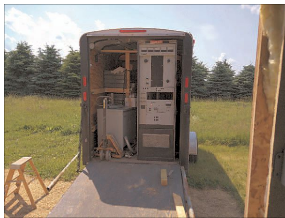
Out With the Old Spare
