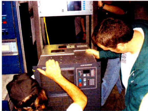
Volunteers install a new transmitter.
