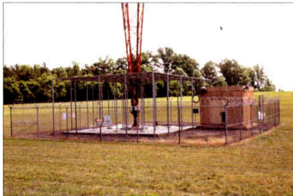
The elevated ground screen "tuned" the vertical radiation.
