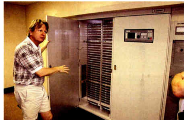
Chief Engineer Jerry Dowd shows off WBT's 50 kW Harris Destiny transmitter.
