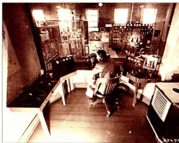
Looking through WGY's Control Room to the Transmitter Room.
