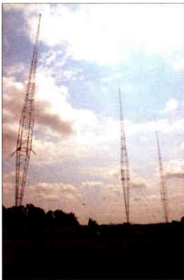
WBT's Directional Antenna is designed to protect KFAB, Omaha.
