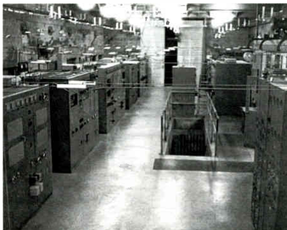
The Press Wireless shortwave transmitters at Belmont, California about 1960.
