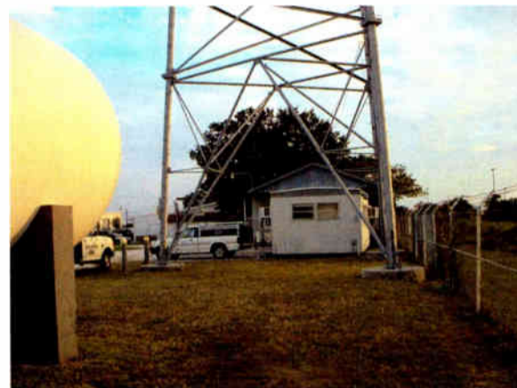
WKZM tower and transmitter building.
