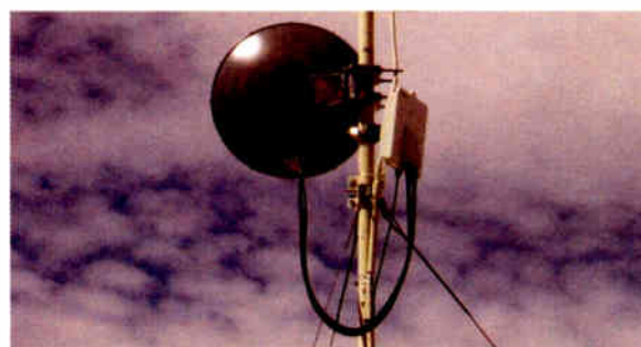
A quick installation and we were ready to go.
