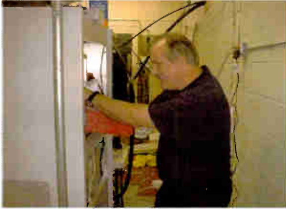
Hard at work cleaning the PA compartment.
