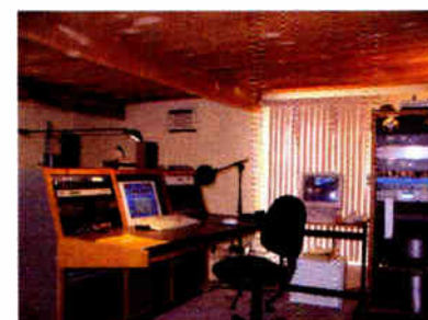
Control A is the On-Air Studio. The STL transmitters, audio pre-processing and EAS stuff are in the rack at the right. Satellite receiver, DigiLink, transmitter remote control and basic production gear is in the Marco console - a video console but quite efficient for this application, and part of our original equipment at KHCS.
