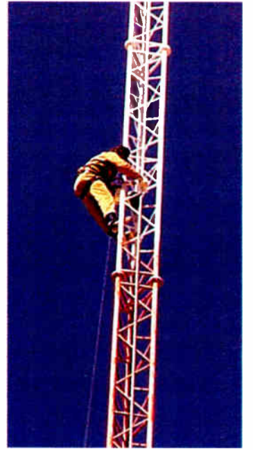
Hire only tower workers who use proper gear.
