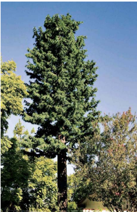
An example of a 50-foot tower disguised as a pine tree. Photo courtesy of Larson Camouflage.
