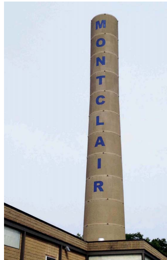
In Montclair, N.J., a fake smokestack goes through one of the sanitation department's historical buildings. The town specified that it had to accommodate a certain number of antennas. Photo courtesy of Stealth Concealment Solutions
