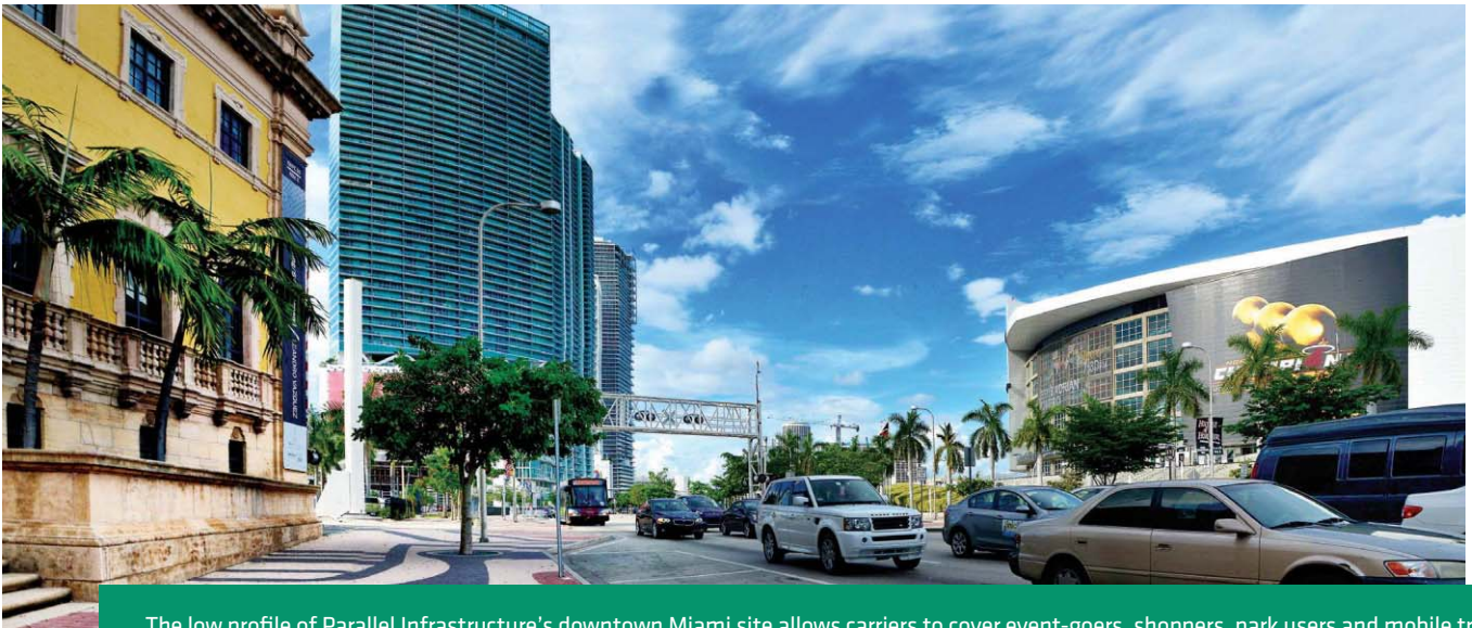
The low profile of Parallel Infrastructure's downtown Miami site allows carriers to cover event-goers, shoppers, park users and mobile traffic.
