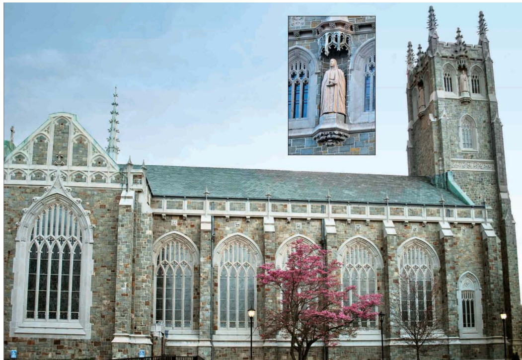
Four sculptures conceal antennas at St. Paul's in Cranston, R.I. Religious sculptures cast in fiberglass are examples of architectural enhancement. Photo courtesy of Environmental Integration
