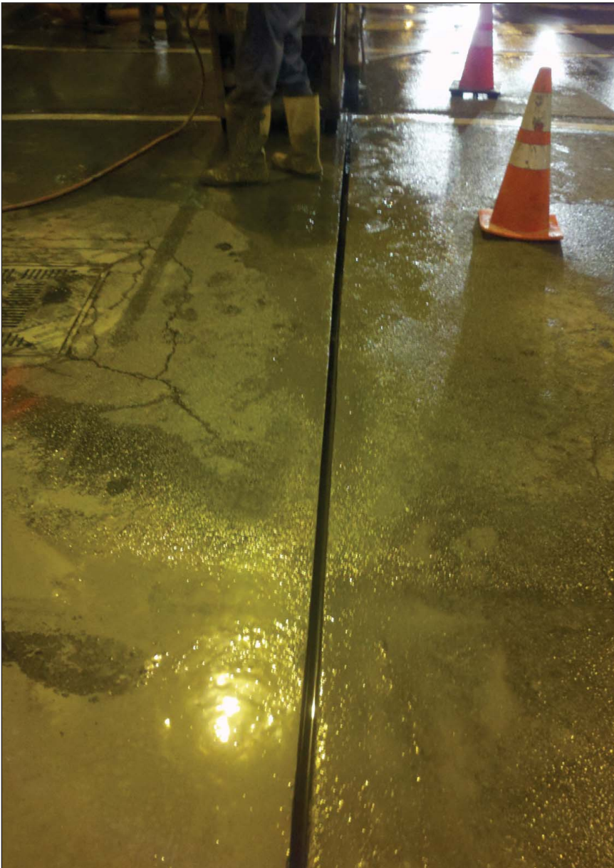
Photo 2. Microtrenching is less time-consuming and invasive, and it allows traffic to pass over the trench line without concern for causing damage. The trench width is usually 1 inch or less, and because less material is removed, it can be easily restored.
