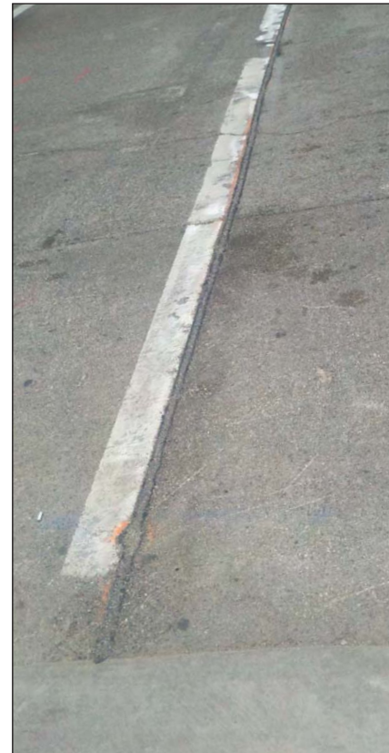
Photo 3. A restored trench appears just to the right of the white line.
