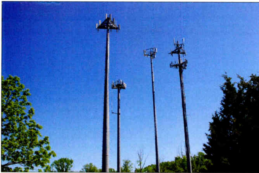
Wireless carriers began using monopoles for a high percentage of their antenna sites as cellular networks saw rapid growth in the late 1980s.
