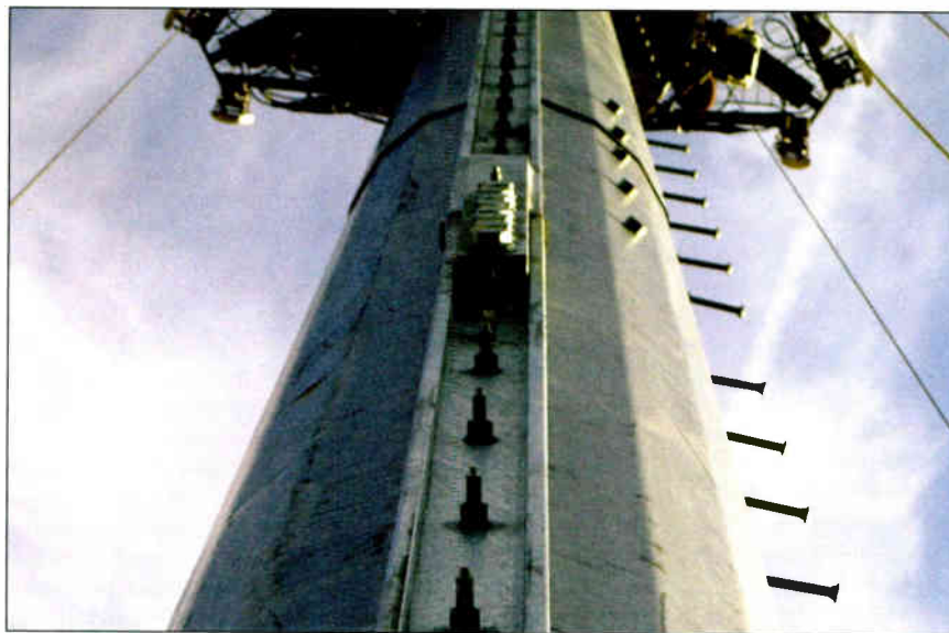
Intermediate-connection blind-bolts are spaced at 18 to 24 inches, depending on the MP3 section used. Bolt spacing is much greater than that required for the equivalent design using flat-plate steel.
