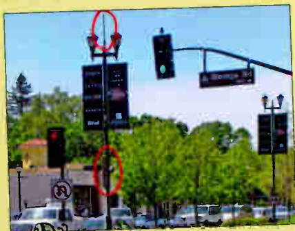
DAS antennas, like the one atop this median lighting standard, can target coverage in urban areas.
