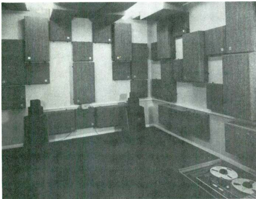
FIGURE 4: KEF auditions its speakers (in this case, a pair of Model 105s) in a specially designed listening room. Sound absorbers on the walls and ceiling help to control reflections and produce conditions for a good stereo image.
