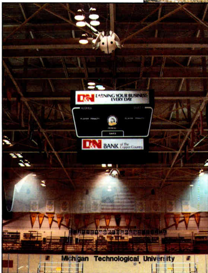
The ice/main floor receives primary sound reinforcement from two Soundsphere 2212-2 speaker systems (above) that each cover one-half of the surface.
