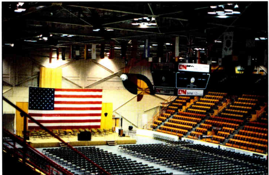
The 34 clusters surrounding the seating areas are each made up of two Community RS-220 speakers. The clusters are spread 25½ feet apart and suspended from a steel grid along the ceiling that runs around the entire room.
