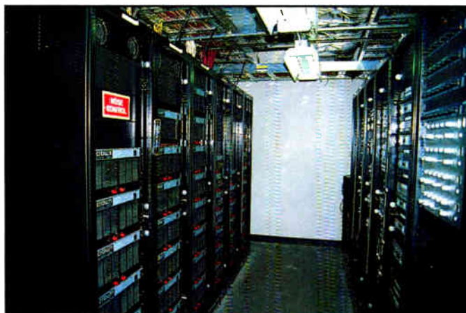
The clusters are powered by 52 Crown Com-Tech 800 amplifiers, while Com-Tech 1600s power the underbalcony and auxiliary systems.
