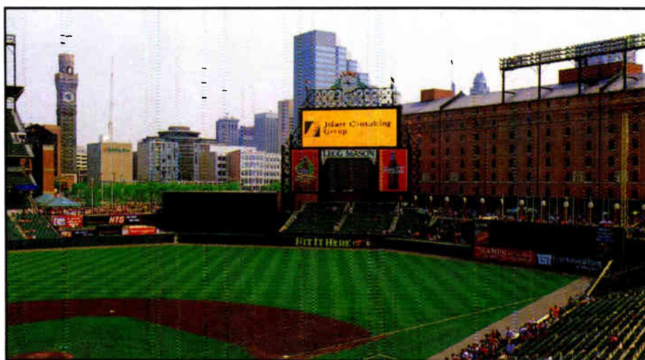
Baltimore's Oriole Park at Camden Yards.
