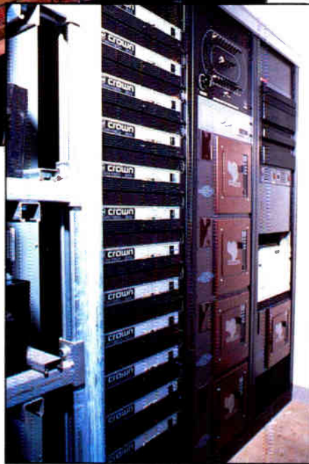
Amplifiers and electronics for the Kezar system are housed in three 72-inch racks located in a structure at the rear of the west end zone. Power is supplied by nine of Crown's Com-Tech 200s and three 400s.
