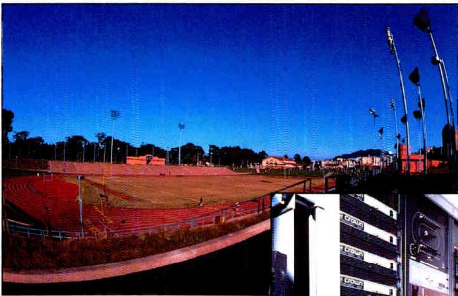
Unlike the former home of the 49ers, the new Kezar Stadium was built entirely below grade, with the tops of the spectator stands extending up to a ground-level promenade.
