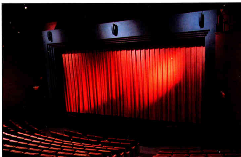
The Chiswick has three Bose 502A Controlled Arrays mounted on the proscenium that allows for stereo music and sound effects program material as well as center localization for actor's voices.
