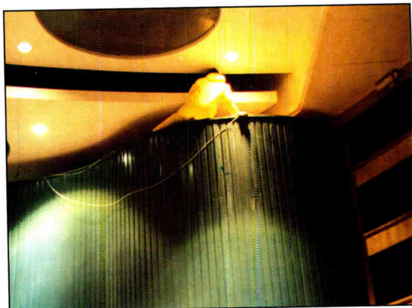
Installation crew in action.
