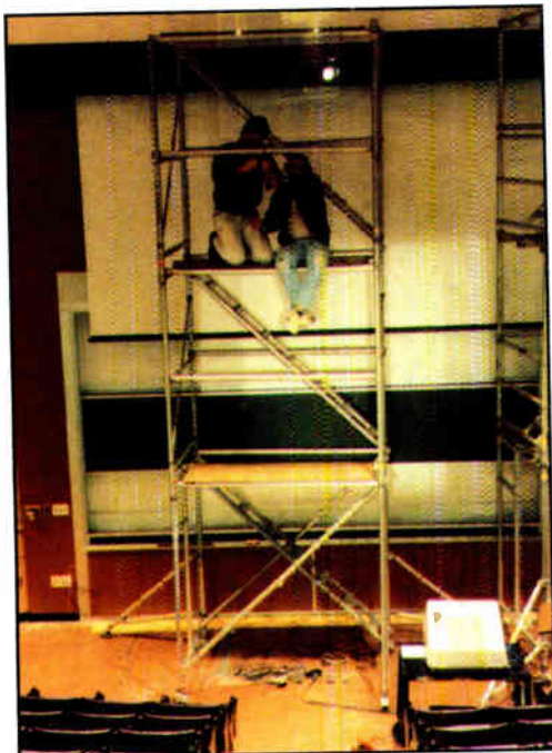
Installation crew installing the mics and baffles.
