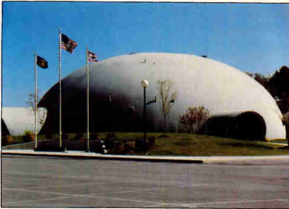
The New Bremen Legion Hall in Ohio.
