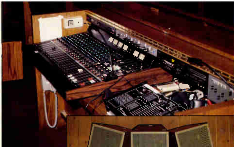
The Yamaha MC1604 console in the chapel (top) and the chapel cluster (right).
