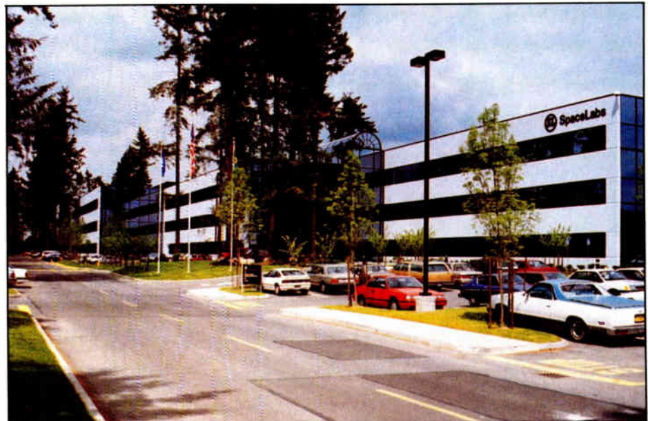
London Controls installed the training rooms and noise masking for SpaceLabs, a medical equipment company.
