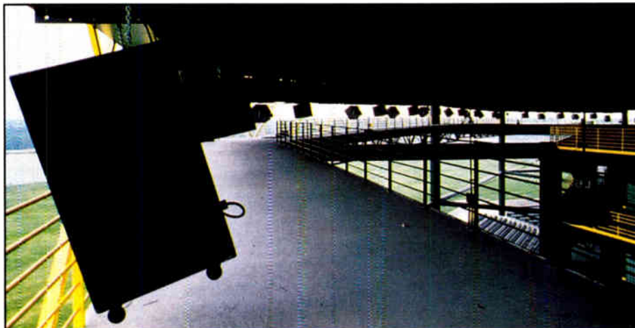
Twenty-six three-way speaker cabinets are used to house four different JBL components.
