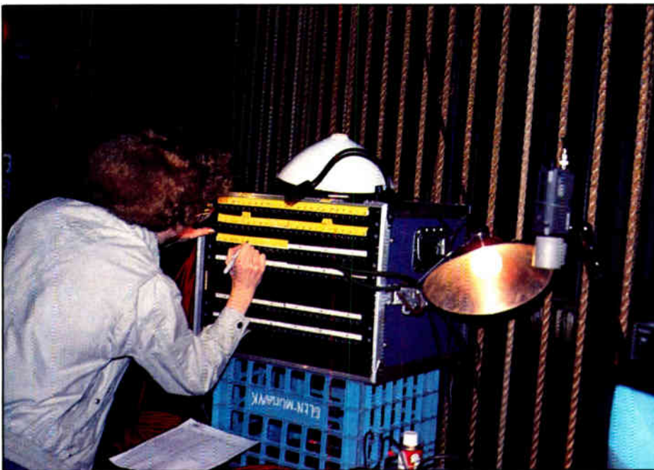
The microphone patch panel is set up in the switching of mic channels for each act. To the right is a CCTV camera pointing downwards a clipboard that gives the numbers of each mic channel.
