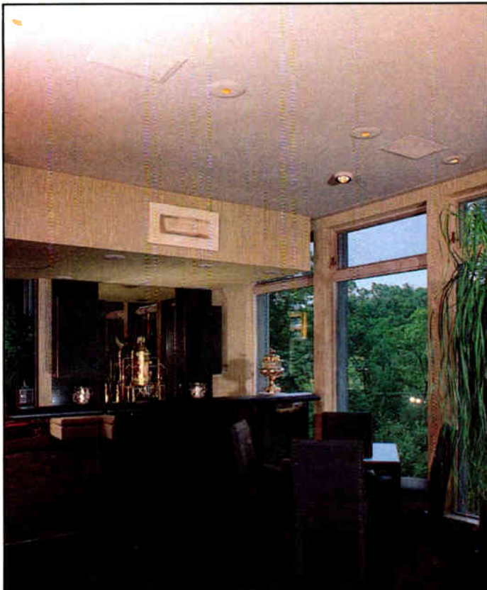
The family room, an independant zone, serves as the primary equipment location (housing the centralized equipment rack) and features four ceiling-mounted Sonance IV loudspeakers, with one M&K V1B subwoofer.
