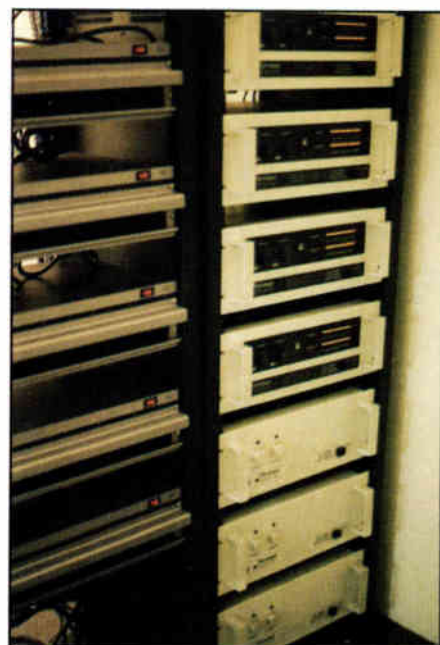
Sound is provided for the main auditorium via [left rack] five SCS 2600 stage monitors and [right] four Perreaux 8000B amps and three smaller Perreaux 600B amps.
