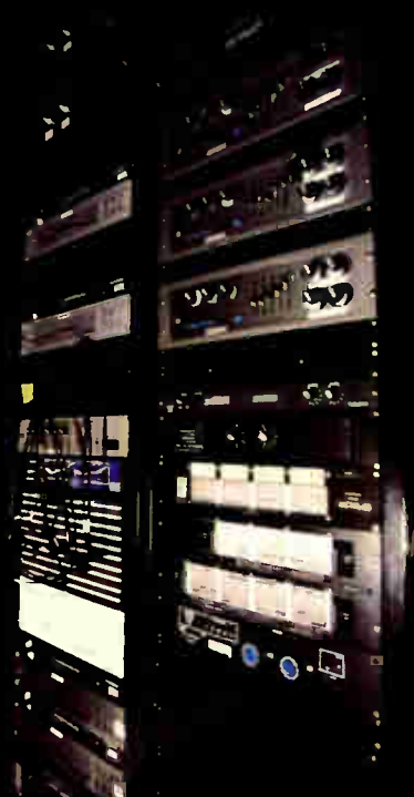
Sound control racks include three Bogen CT 100 monitor amps and a Lexicon Model 92 digital delay unit.
