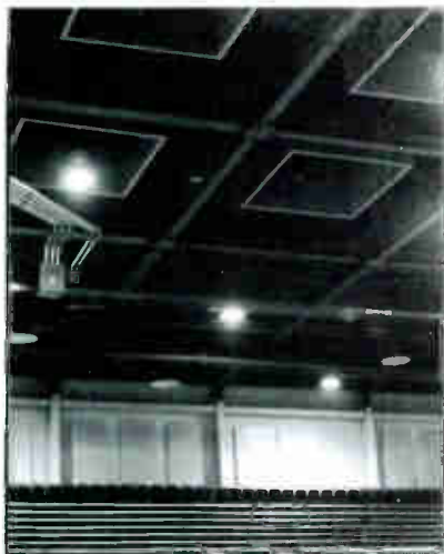
Varitone Sound-Absorbive Modules are attached to the sidewalls and suspended in squares from the ceiling in Hall A of the Washington (D.C.) Convention Center. The modules reduced the reverberation time in the hall from 6.4 seconds to 2.9 seconds.
