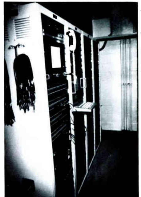
Manatei Civic Center's control room.
