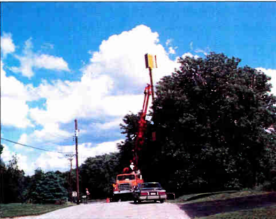
The crew sets up the completed WS-3000 system.
