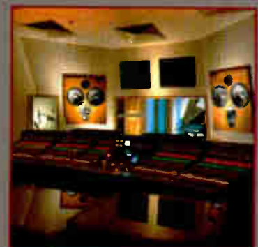
The Gallery Control Room
